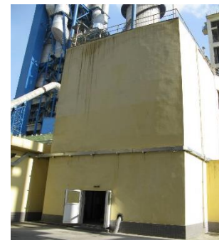
Photo: Sludge storage silo
